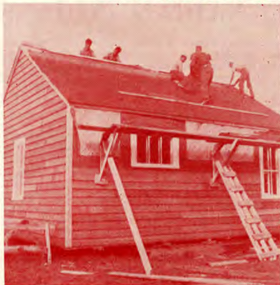
House under construction by the Joussard I.R.S. Manual Training Pupils.
